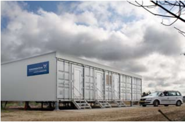
Figure 1. - Full-scale modular MBR-based wastewater treatment plant - Bjerregrav, Denmark
