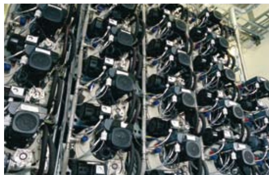
The 23 PBRs are installed in vertical layers to ensure max. compactness and flexibility in case of future expansions.
