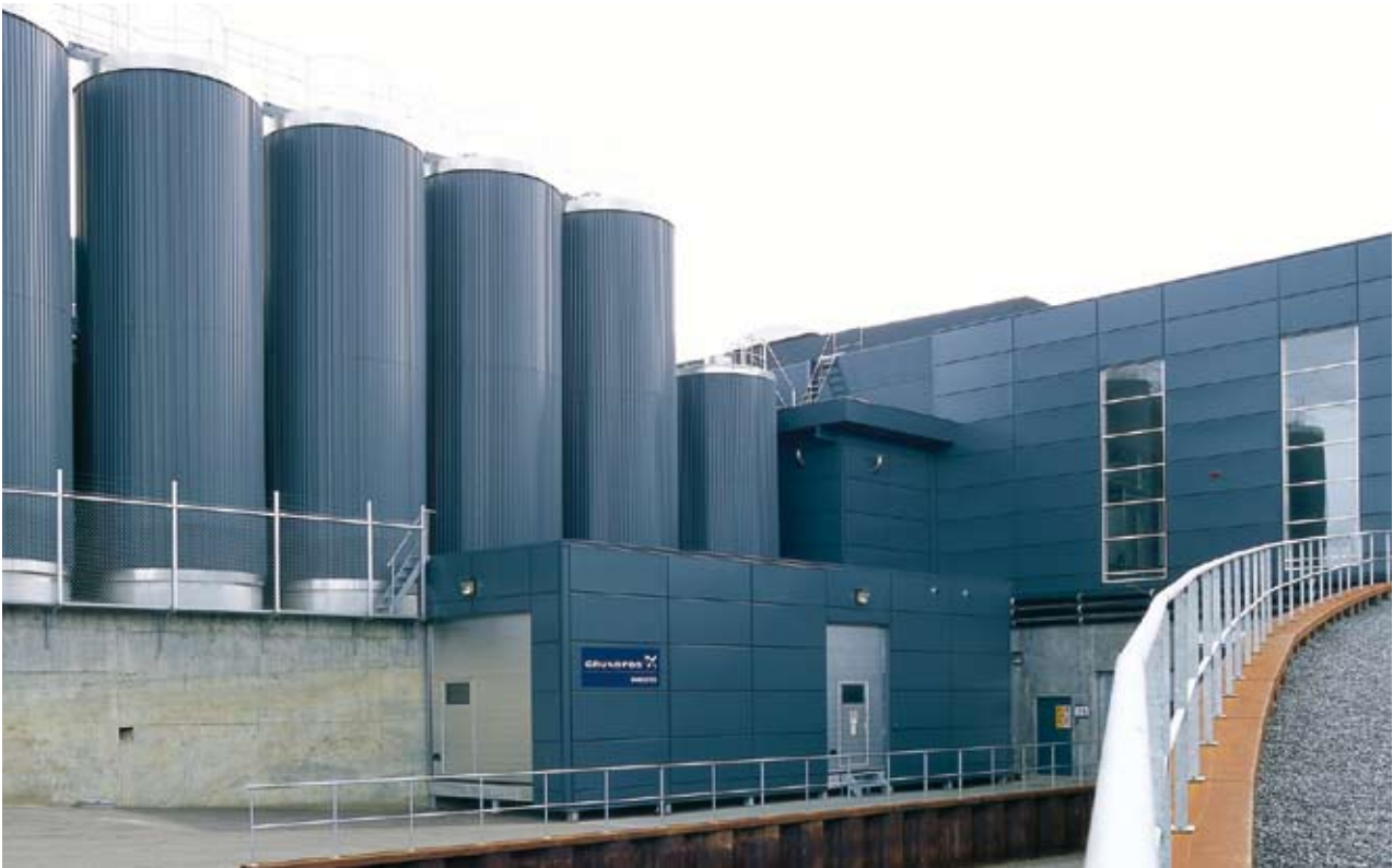
A 62 m 2 building accommodates the complete BioBooster plant!
